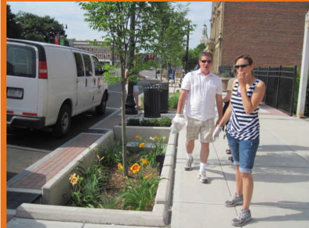
Pittsfield's streetscapes program includes creating stormwater planters with trees, within the right of way.
