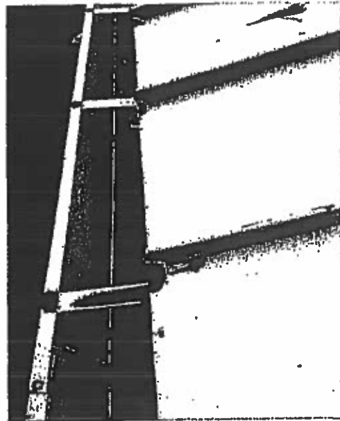
The badly deteriorated gutters were repaired (temporary) with a combination of new metal and rubber seal and stick material. Full replacement of the gutter system is recommended.
