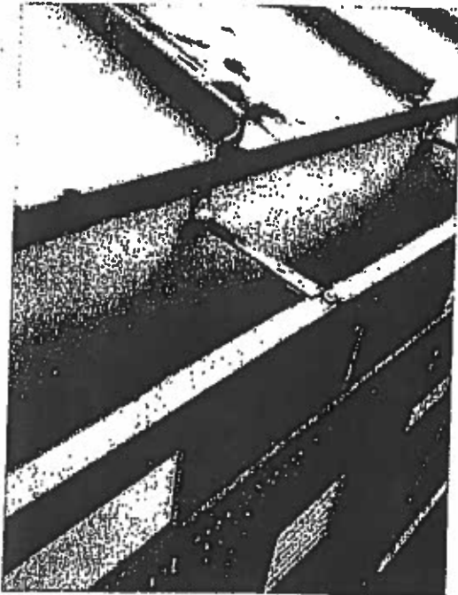
The badly damaged gutter on the west side of the facility was re-attached and repaired. The missing downspouts found on site were reinstalled during the project.
