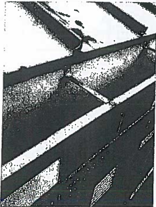
The badly damaged gutter on the west side of the facility was re-attached and repaired. The missing downspouts found on site were reinstalled during the project.
